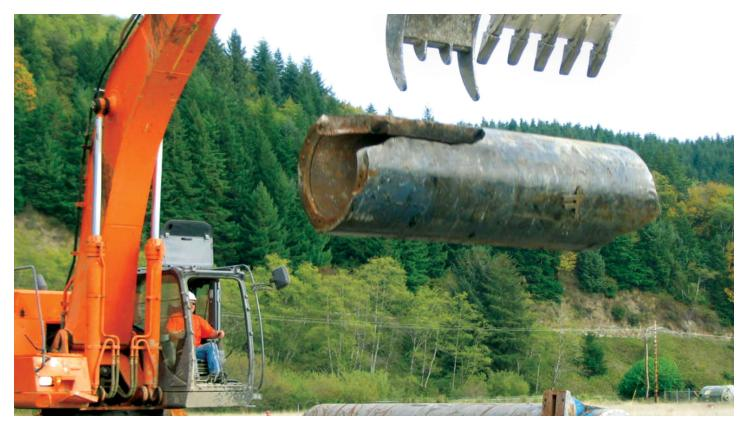
A cut piece was used to drop on to the remaining three pins to break them into pieces small enough to be carried away.
