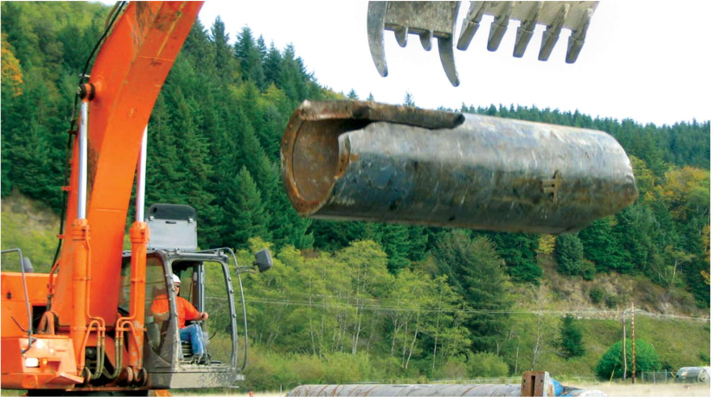
A cut piece was used to drop on to the remaining three pins to break them into pieces small enough to be carried away.
