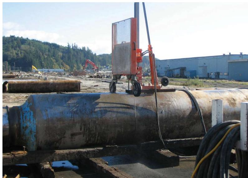
The wire saw was used to cut half way through the steel rolling pin.
